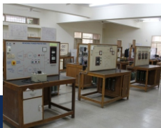
Power System Lab
